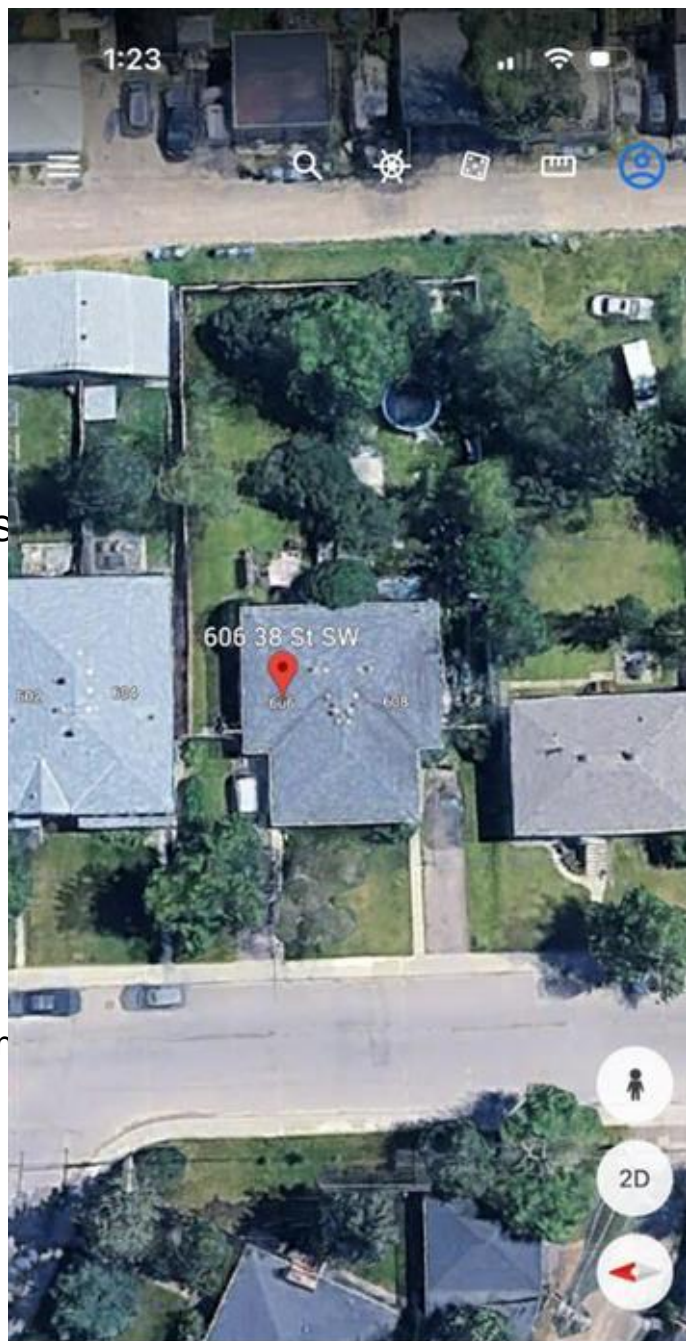
606 38 St SW Building
